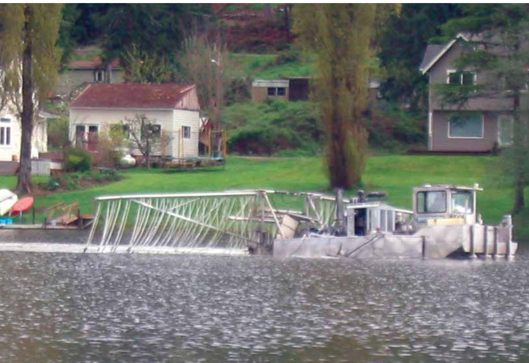
Figure 4. Alum application Long Lake, Kitsap County, Washington, April 2007.
